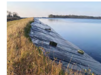
2. HDPE membrane lined reservoir
