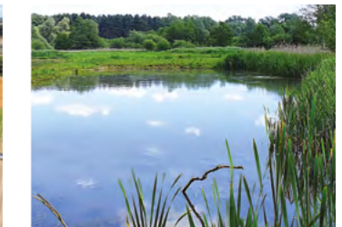
4. Finished integrated reservoir
